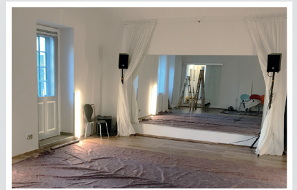
Moisture protection at the studio
